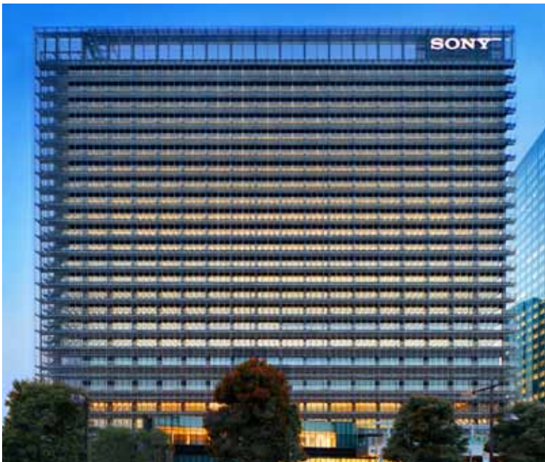
Figure 6: Every expenditure of carbon through the embodied energy in materials and systems needs to be justified by overlaying more usage on those systems. In the 2011 NBK Osaki Building in Tokyo, the “Bioskin” solar shading shields internal spaces from solar gain and, through the system containing recycled rainwater, simultaneously reduces the external urban heat island effect through evaporation. Copyright: Nikken Sekkei
