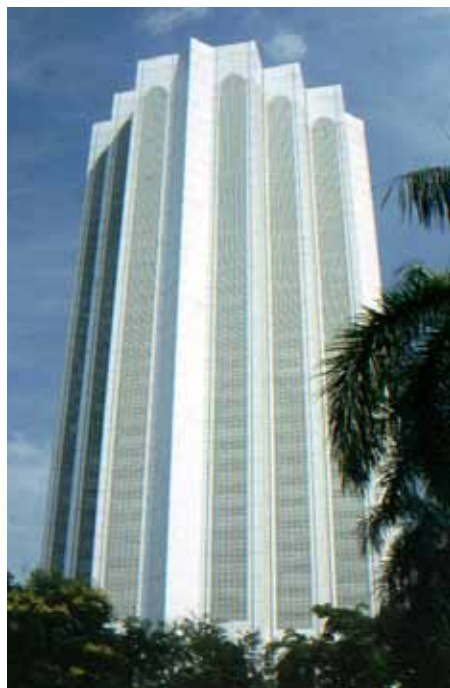
Figure 4: Tall Buildings can reflect the local culture in a literal way – as demonstrated here with the 1984 Dayabumi Complex in Kuala Lumpur with its façade a modern interpretation of the Islamic jali screen – or in a more direct way, by incorporating specific activities and ways of life into the program of the building. Copyright: Antony Wood
